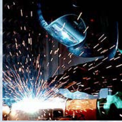
welding & construction works
